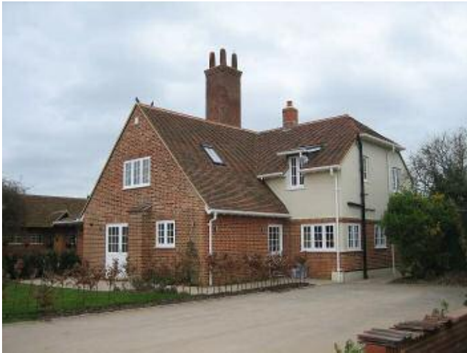
The Pump House today
