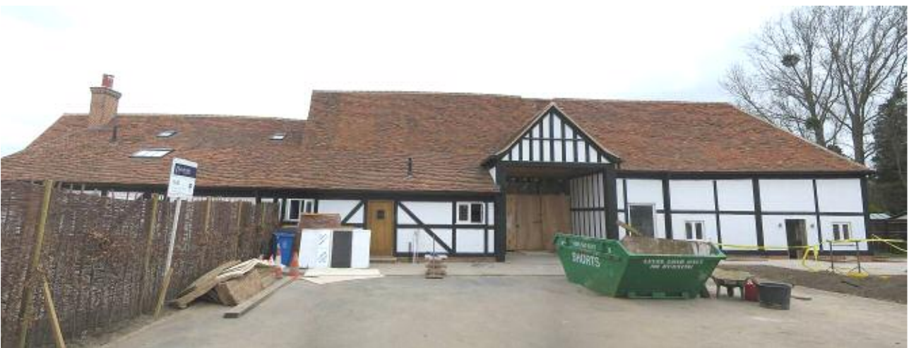
.....and restoration nearing completion
