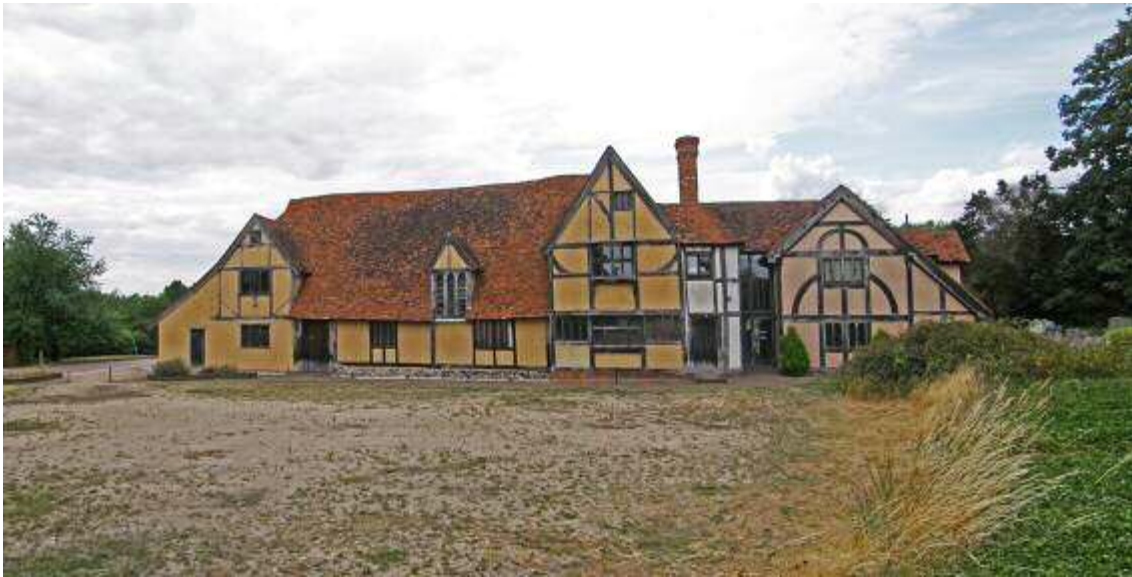
Upton Court – a 14 th century building with a 20 th century annexe
