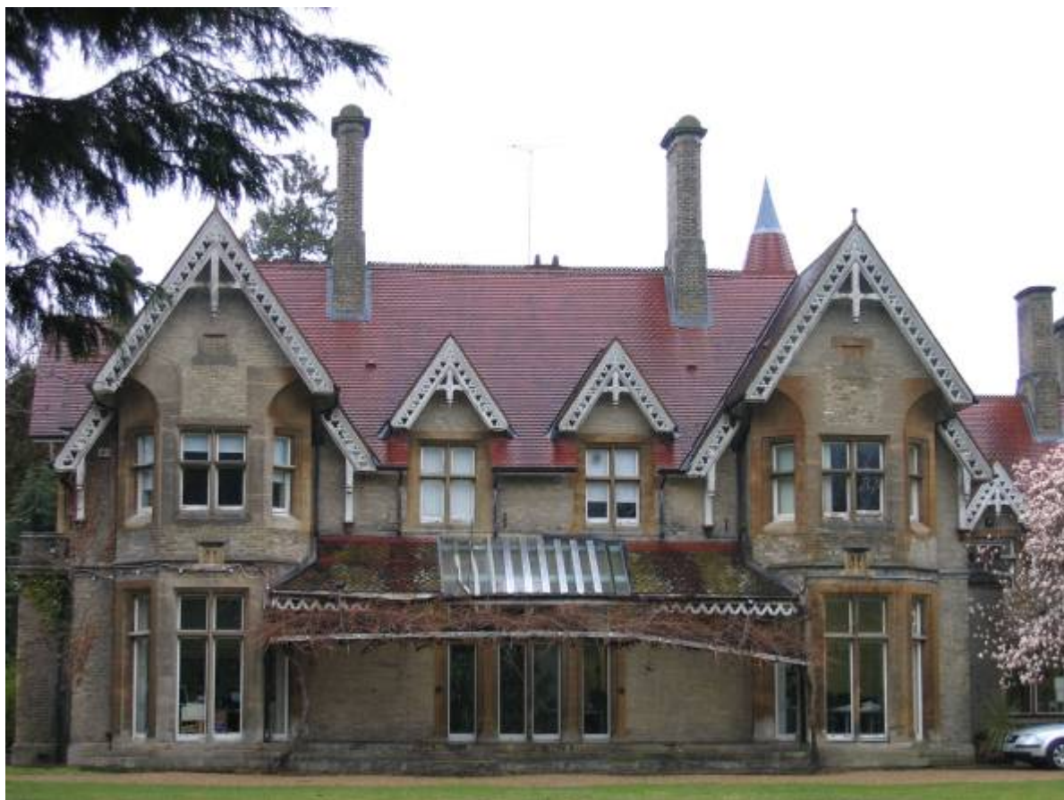
Glen Island House, built in 1869
