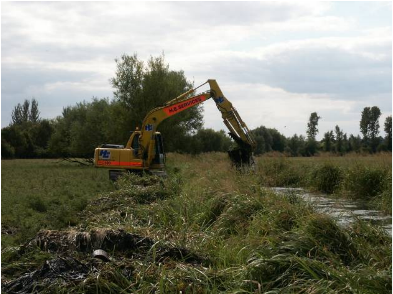
Digging out the White brook on Widbrook Common
