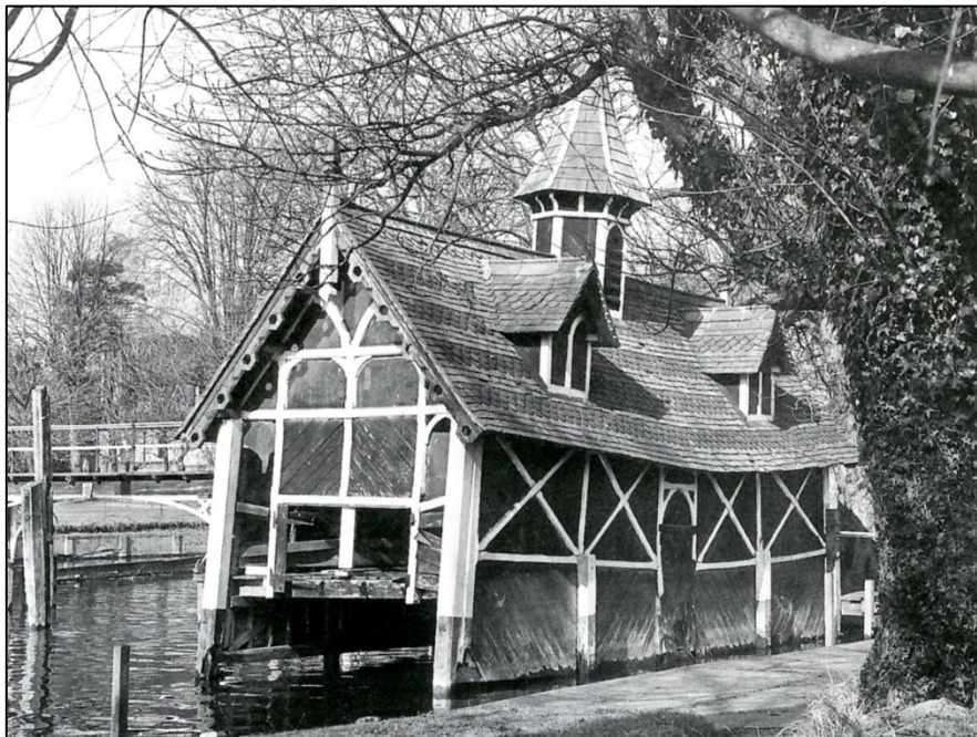
The derelict boathouse not long before its almost complete collapse
