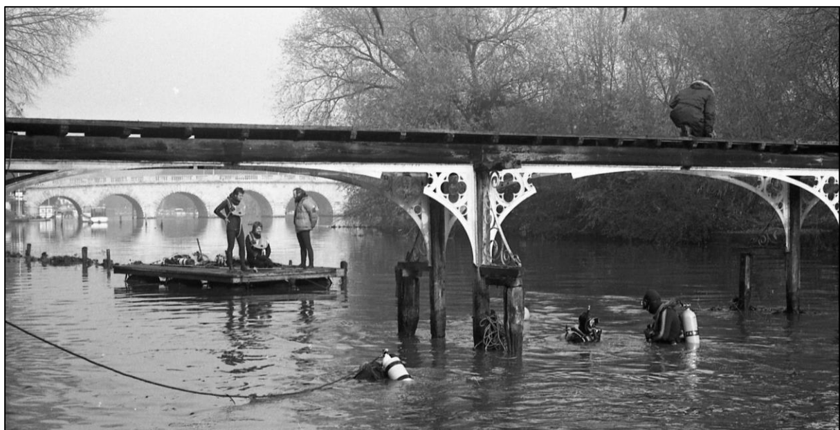
Divers inspect the foundations of the decaying bridge
