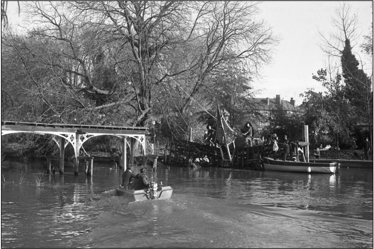
Maidenhead scouts get ready to lift off the boathouse spire.....
