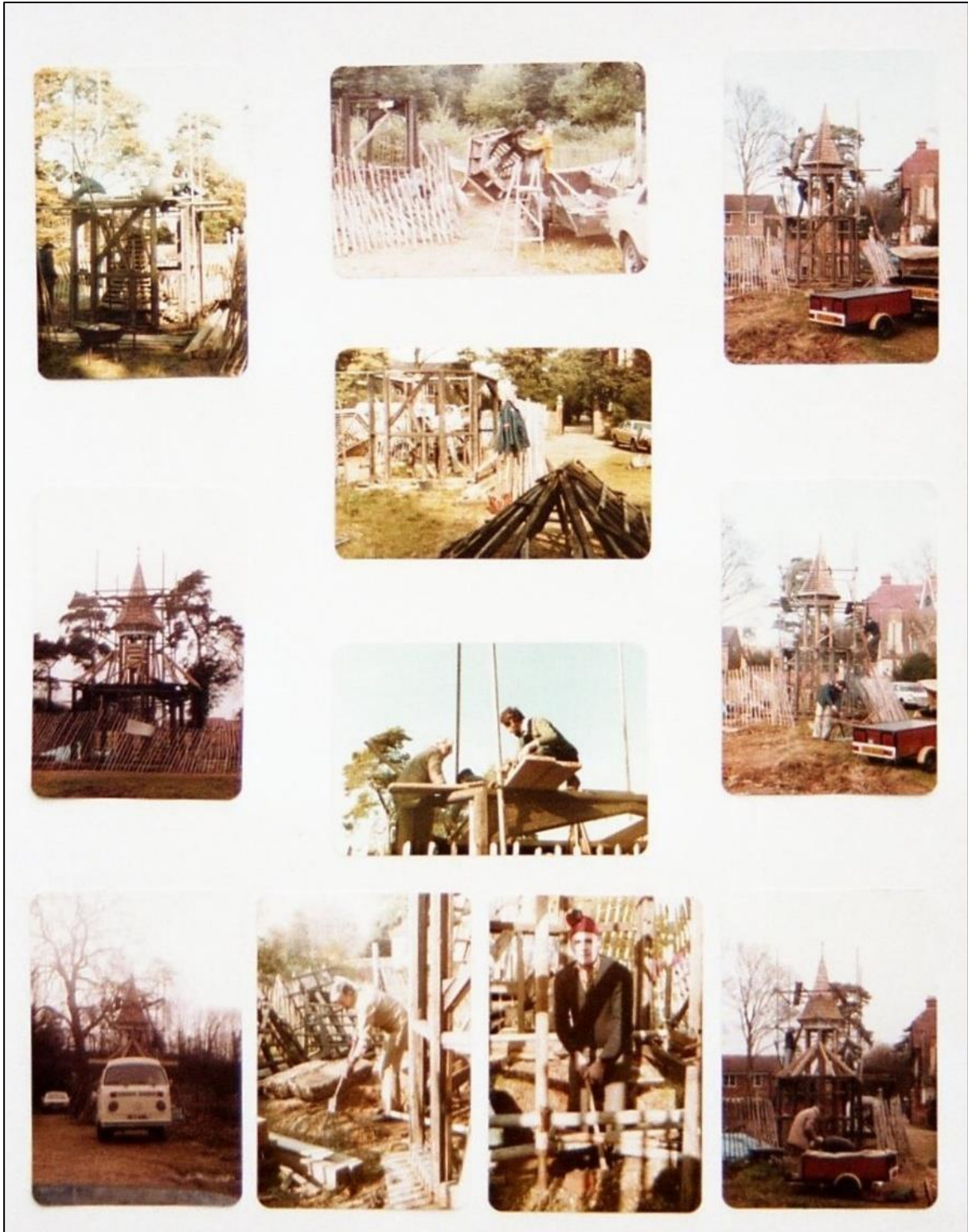
A montage of photos, assembled in 1989 for the exhibition accompanying the unveiling of the commemorative plaques, showing various stages in the construction of the shelter. Unfortunately the originals are now lost
