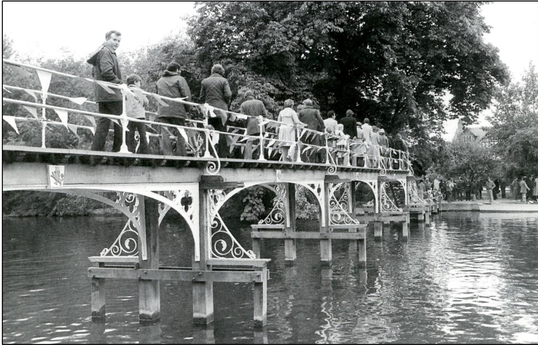
The bridge open at last to the public – their first chance to walk over to the island
