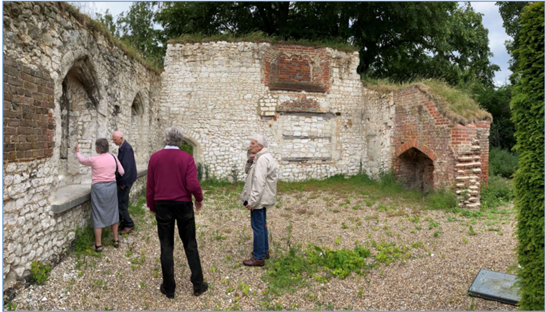
Society members inspect part of the original C13th building
