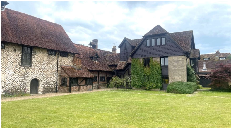
Michael Bayley modified the newer building to the right of the photo
